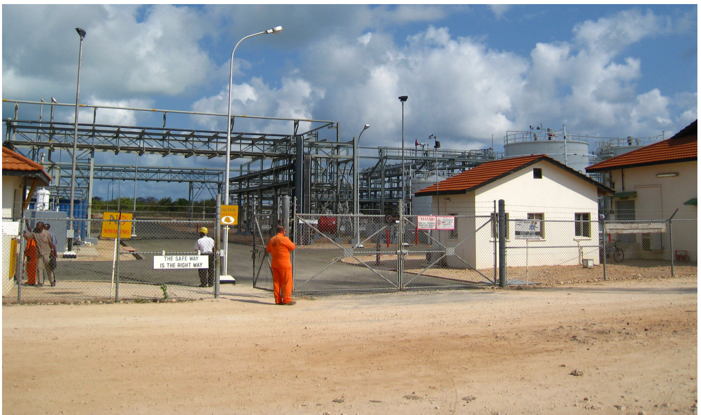
Songo Songo Gas Plant
